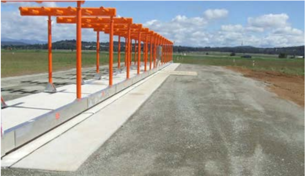
Figure 2.1: Typical Localiser Installation
